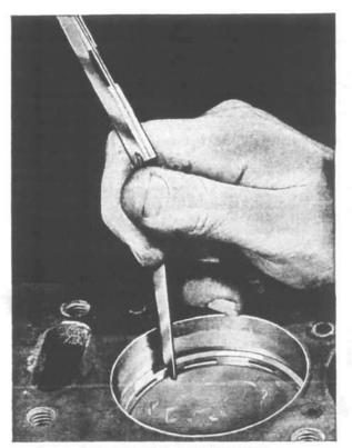
FIG. 116-PISTON RING GAP
