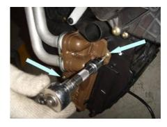
4.1.4. Remove the two screws on front end of hot water pipe with cross screwdriver.
